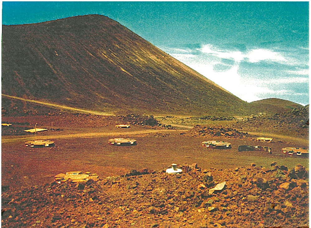
Submillimeter Array antenna pads--10 feet each in diameter, scattered over an area of about a quarter mile wide.
