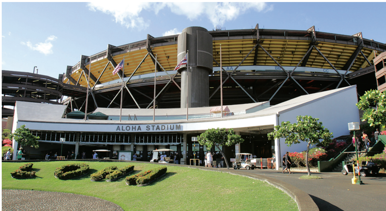
PHOTO: ALOHA STADIUM
