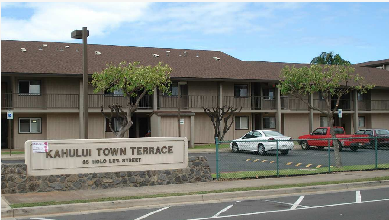
Kahului Town Terrace 72-unit preservation in Kahului, Maui financed with a combination of State and Federal Low-Income Housing Tax Credits, Hula Mae Multi-Family and Rental Housing Trust Fund Loans administered by the HHFDC.
