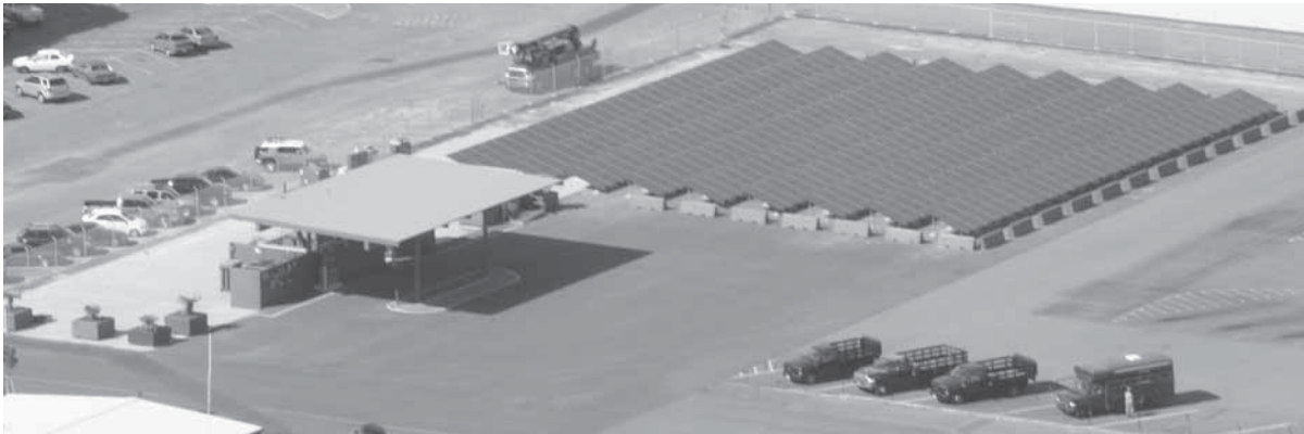
Renewable hydrogen production and fueling station at Joint Base Pearl Harbor-Hickam
