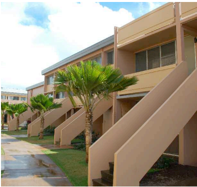
Kukui Gardens HHFDC administered federal ARRA Tax Credit Assistance Program funds for the rehabilitation of 389 rental units in 2011.
