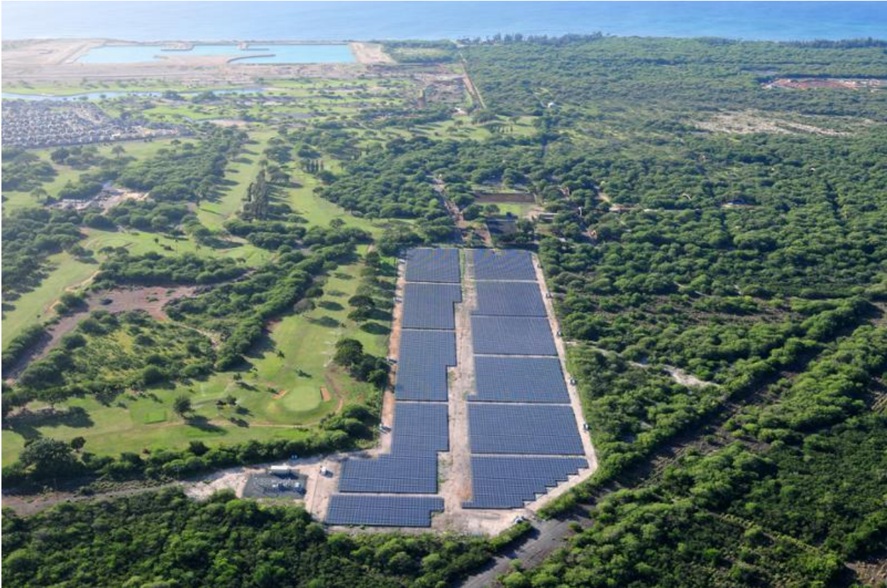
Kalaeloa Renewable Energy Park – Hanwha Solar Energy America (Kalaeloa, Oahu)
