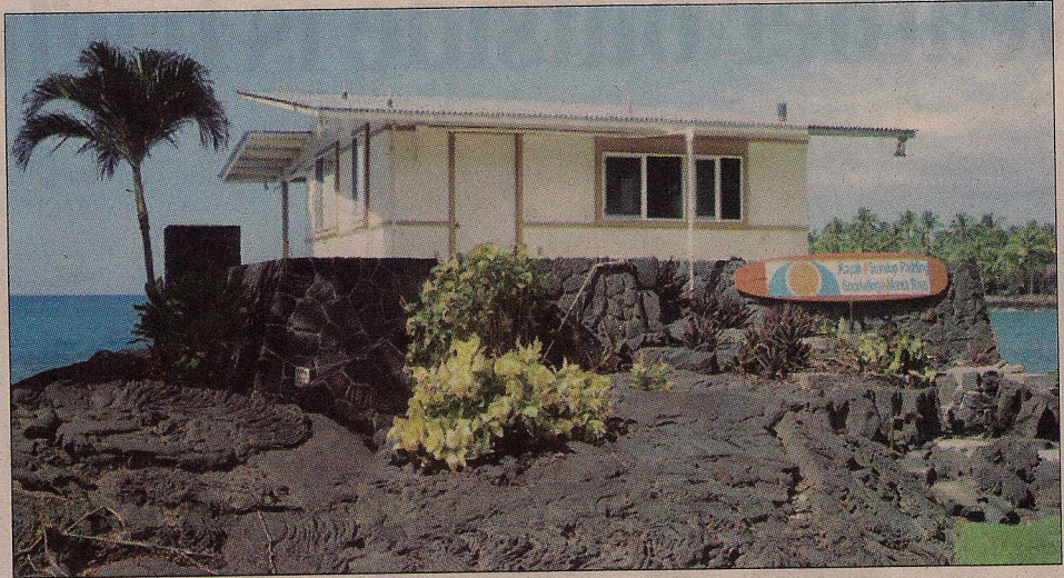
Unpermitted work was also done on this structure at the resort.
