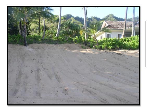
Sand pushing in the summer of 2006, the bulldozer tracks in the sand show the sand that was taken from the beach and pushed mauka to cover the sandbags.
