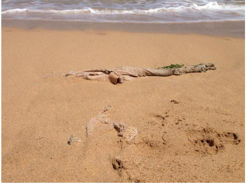
Over the years, the sandbags break apart, littering the beach, reef and rocks, get repaired and replaced and fail again.
