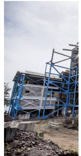
Construction on Hu Honua Bioenergy plant is shown
