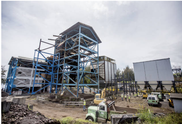
Construction on Hu Honua Bioenergy plant is shown in this August 2017 file photo. (HOLLYN JOHNSON/Hawaii Tribune-Herald)
