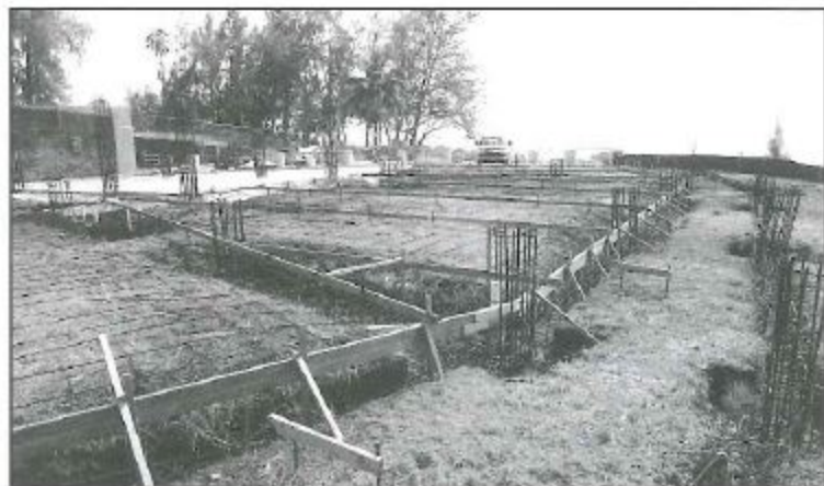
The line of rebar at the right of the photo marks the outer limit of the planned lanai area of the "Pepe'ekeo Palace." Without the public access route being changed, the lanai encroaches into the public access easement running in front of the house site.
