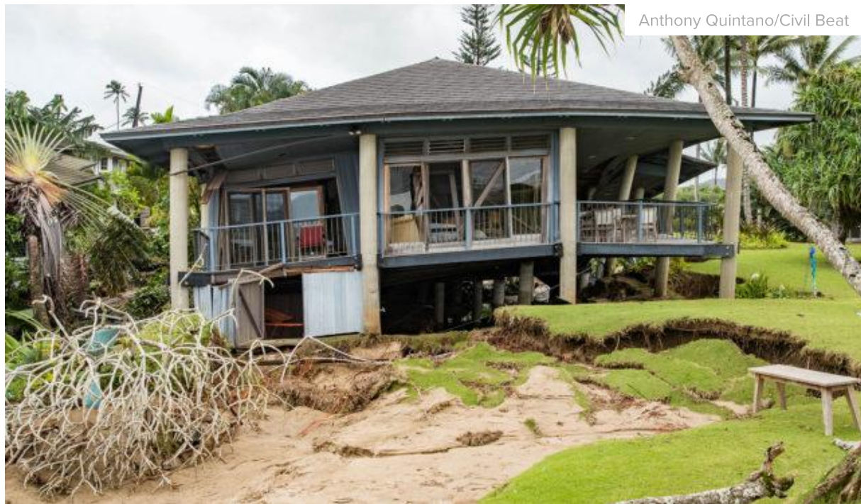
A home along Hanalei Bay's shoreline that was pushed off its stilts by floodwaters.
