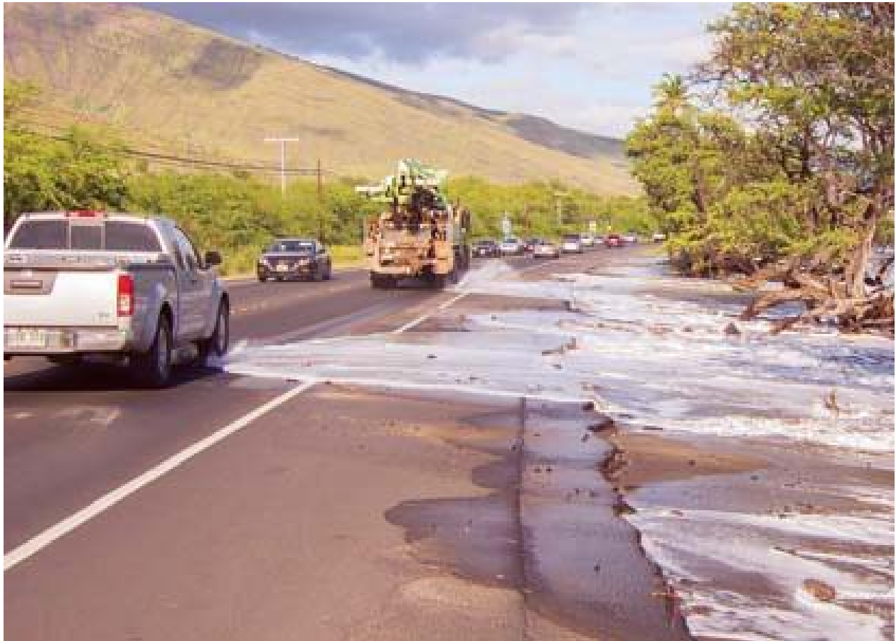
Waves wash over Honoapiilani Highway at Mile Marker 14 in May 2017 in Olowalu. ASA ELLISON photo
