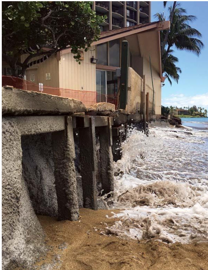
This photo from May 2016 shows erosion threatening a structure and part of Royal Kahana's pool deck. TARA OWENS photo
