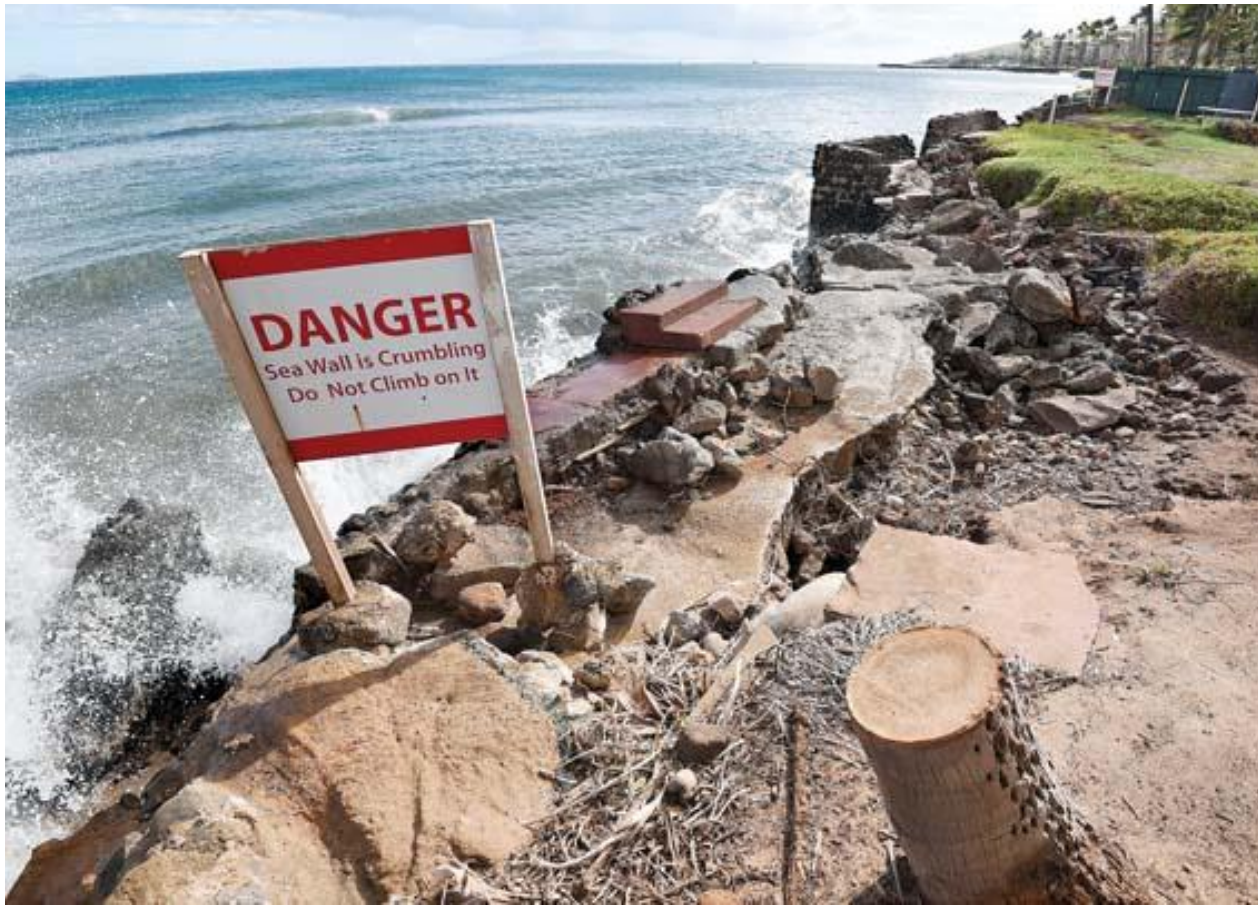
A sign warning about the dangers of a crumbling Maalaea seawall rocks in the wind as its supports are also being eroded.
