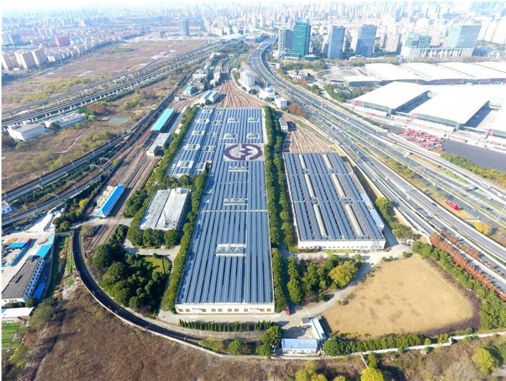
Shanghai Metro Rooftop Solar
