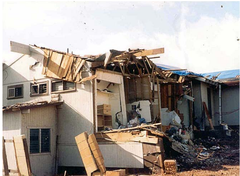
Figure 3: Damage by Hurricane 'Iniki in Puhi, Kaua'i, 1992
