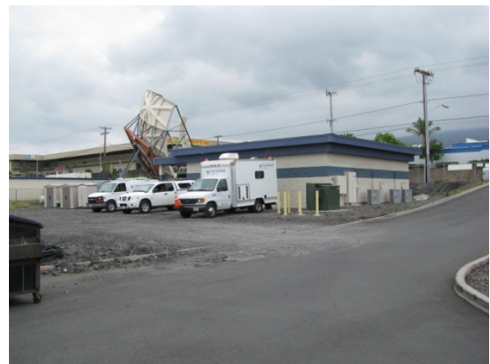
Figure 1: Headend Building in Kona
