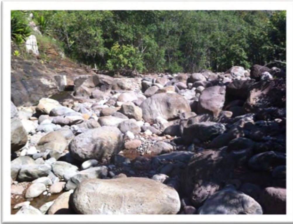
Below Koai'e Dam (outlet at left)
