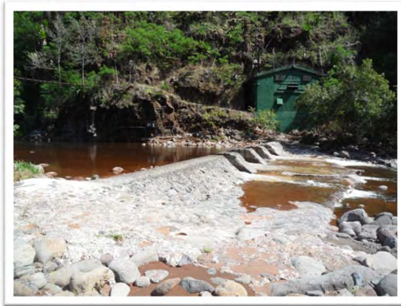
Mauka Powerhouse Dam
