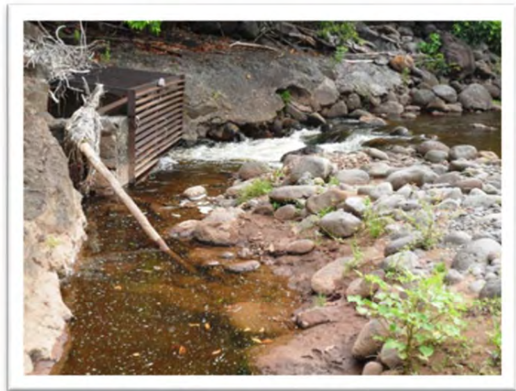
Koai'e diversion, looking from top of dam
