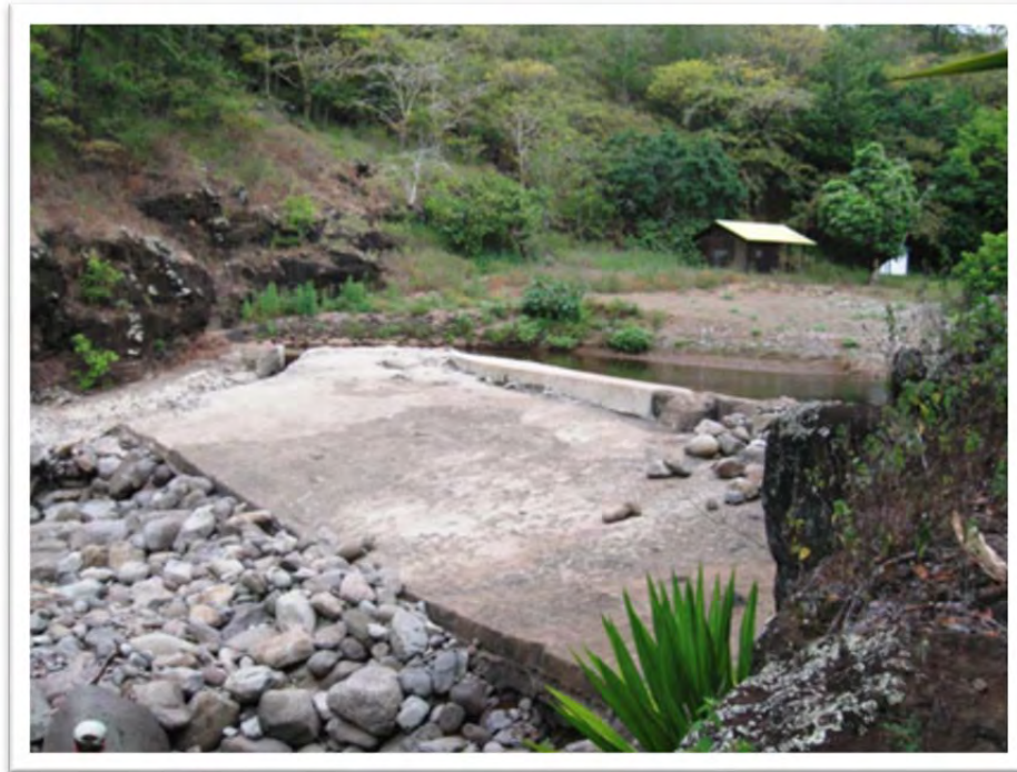
Waiahulu Dam, view from east
