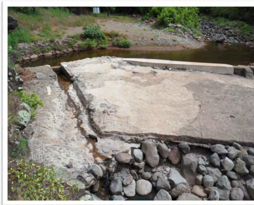
Waiahulu Dam (boarded-up outlet in middle left)
