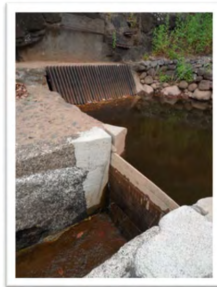
Waiahulu Dam diversion grate and boarded-up outlet
