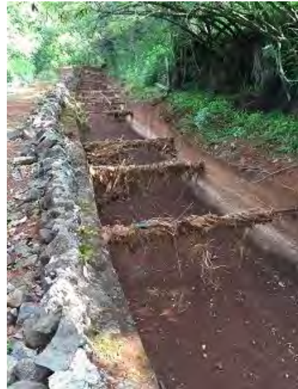
Photos of sediment accumulated within KEDIS resulting from August 25, 2015 storm runoff
