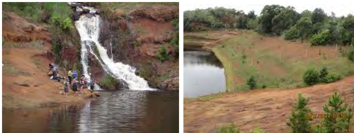
Kōke'e Ditch Entering Pu'u Lua Reservoir; Exposed Reservoir Height Staff Poles
