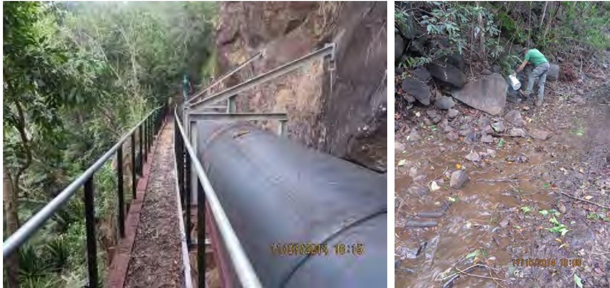
Long Section of HDPE Installed to Replace Original Wooden Flumes and Leakage Along Road
