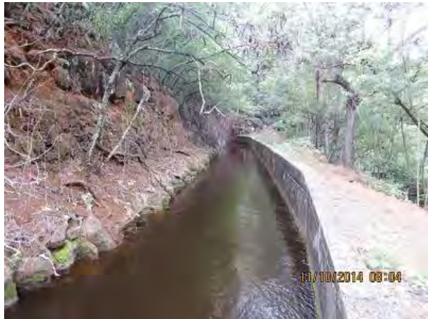
Storm Water Diversion Structure on KEDIS; Recently Lined Leaky Ditch Section Before Tunnel 7
