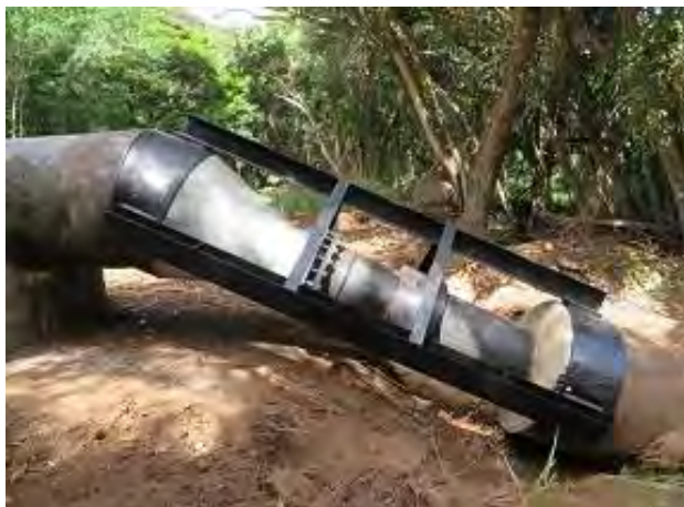
Top of Black Pipe Siphon; Reduced Diameter Liner Pipe Installed in Black Pipe Siphon
