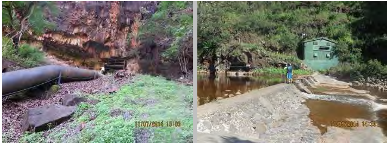
Penstock and Fore Bay at Tunnel Exit; Mauka Hydropower Plant and Original Waimea Ditch Inlet
