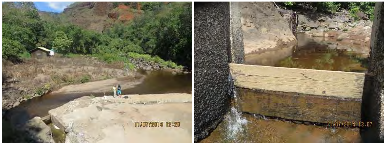
Wooden flashboards in spillways in dams on Waiahulu (lower left of photo) and Koaie streams
