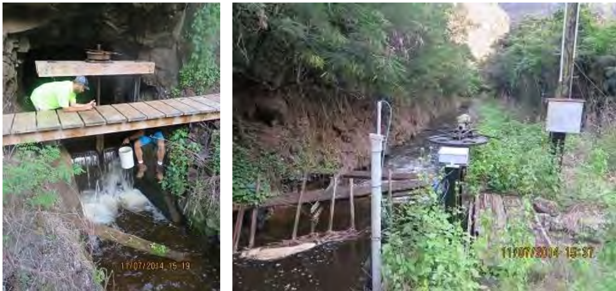
Upper and Lower Diversion Points Located Just Below the Mauka Hydropower Plant
