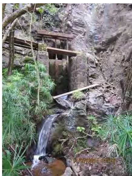
Leakage from Secondary Diversion and 0.61 mgd Streamflow below Upper Intakes of KEDIS
