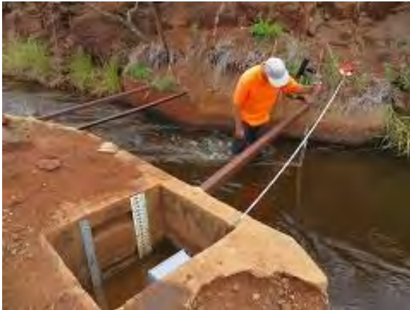
Measuring Ditch Flow at Hukipo Flume on KEDIS; Typical Unlined KEDIS Section
