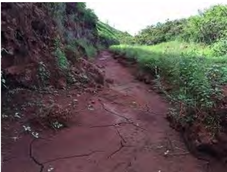
Photos of sediment accumulated within KEDIS resulting from August 25, 2015 storm runoff
