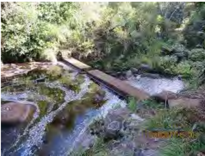
Diversion Dam on Kaua'ikananā Stream and Diverted Flow Entering Tunnel Below Dam
