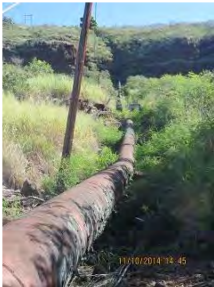
Penstock Leading to Waiawa Hydropower Plant; Water Exiting Waiawa Hydropower Plant
