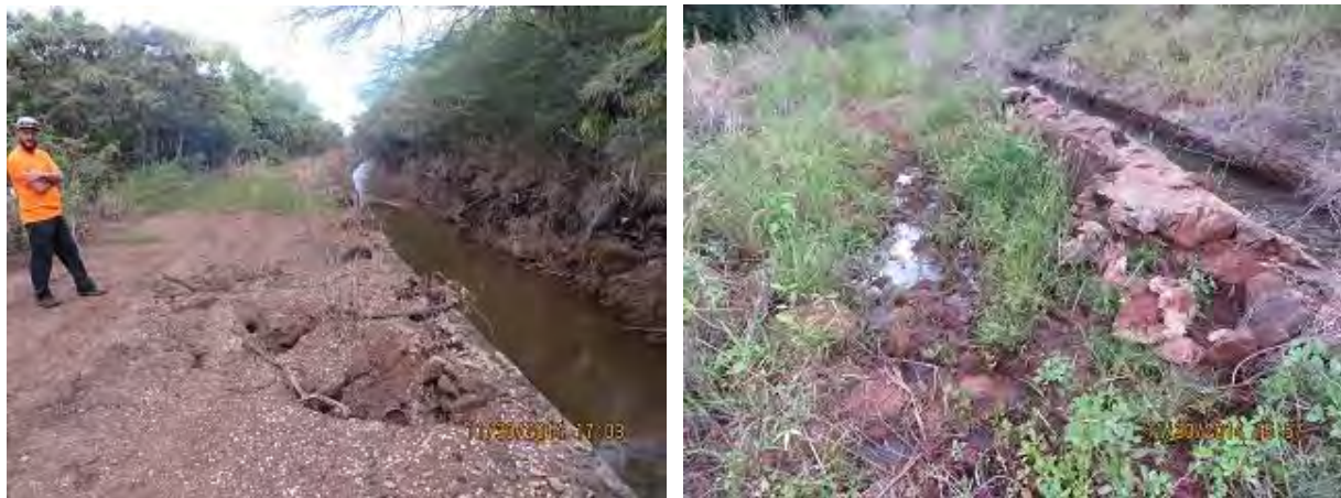
Collapse Features and Leakage Below Walls of Lower Section of KEDIS
