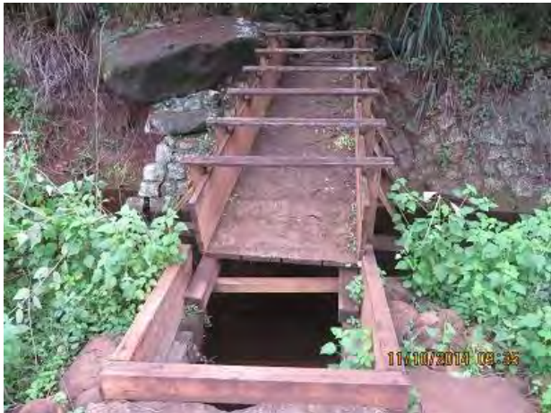
Storm Water Diversion Structure on KEDIS; Recently Lined Leaky Ditch Section Before Tunnel 7
