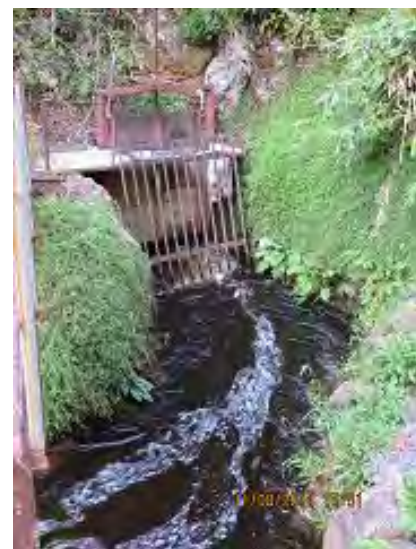
Diversion Dam on Kaua'ikananā Stream and Diverted Flow Entering Tunnel Below Dam
