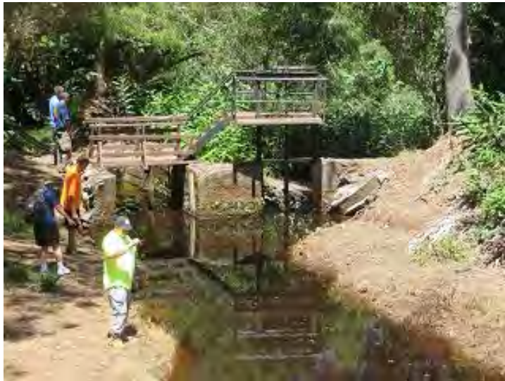
Kauhao Diversion Structure; Ditch Water Leaking Under Flashboards at Kauhao Diversion
