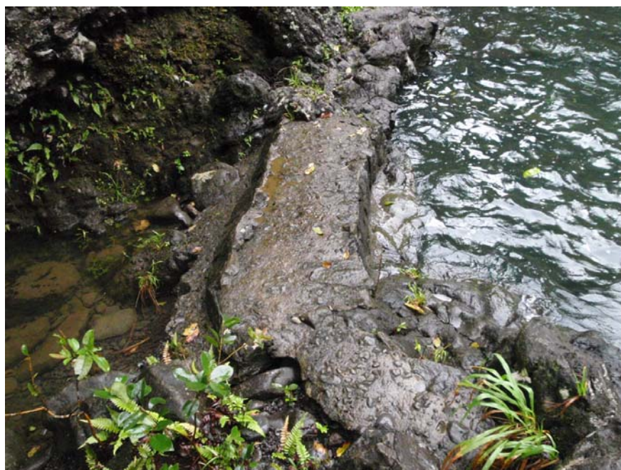
Figure 5-19. Photo of concrete wall damming water for diversion intake above survey site 3. (3/9/2009; Tributary name: Waiohue (64018001); PBN: sh003p-016-030909; Surveyor: Hau, S.; Habitat type: Pool; SBN: sh003r-030909; Lat. (DD): 20.81567, Long. (DD): -156.12628).
