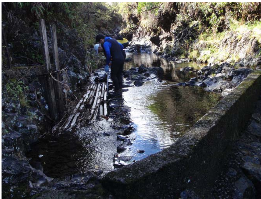
Figure 4-3. Concrete weir next to survey site 6. Photo is taken in the upstream direction. (2/11/2009; Tributary name: Kapā'ula (64021001); PBN: ts006p-123-021109; Surveyor: Shimoda, T.; Habitat type: Riffle; SBN: ts006n-021109; Lat. (DD): 20.80955, Long. (DD): -156.11530).
