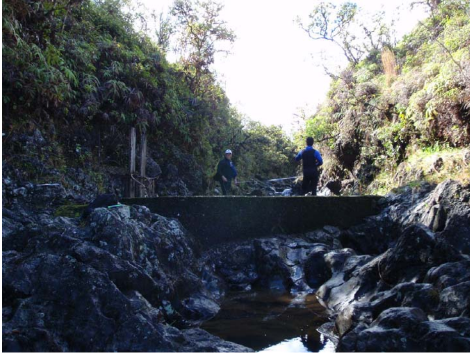
Figure 4-4. Photo is looking upstream towards the survey site 6 and the diversion. (2/11/2009; Tributary name: Kapā'ula (64021001); PBN: ts006p-124-021109; Surveyor: Shimoda, T.; Habitat type: Riffle; SBN: ts006n-021109; Lat. (DD): 20.80955, Long. (DD): -156.11530).
