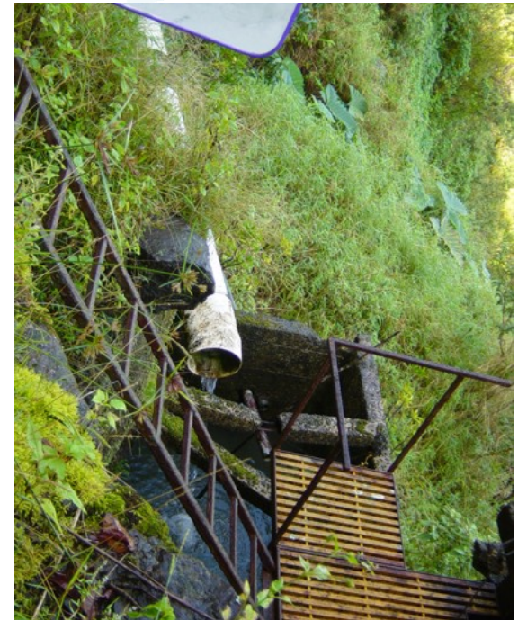
EMI minor diversion that is dropping seepage water into a catchment basin, Waiokamilo Stream
