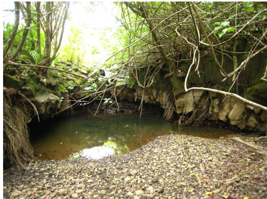
Section downstream of Dam 3
