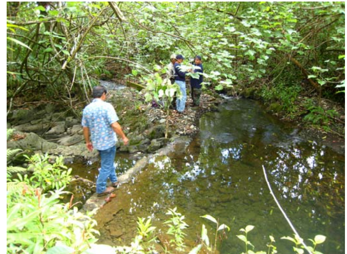
Dam 2 at Waiokamilo Stream, diverting water into the Lakini auwai system
