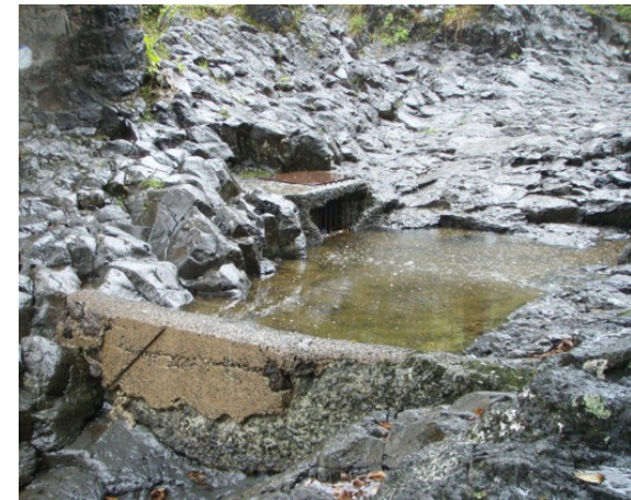
EMI diversion at Koolau Ditch, Piinaau Stream
