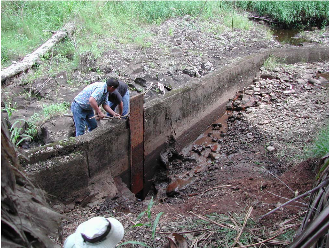
Sluice gate opening is 17-in(W) x 14-in(H)
