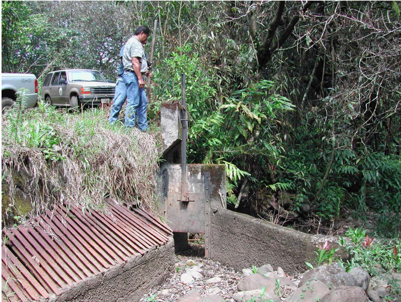
Sluce gate opening is 2-ft(W) x 1.37-ft(H)
