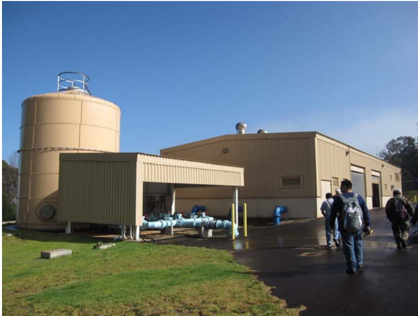
Olinda Water Treatment Facility
