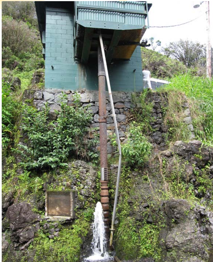
Nahiku Pump on Hanawi Stream
