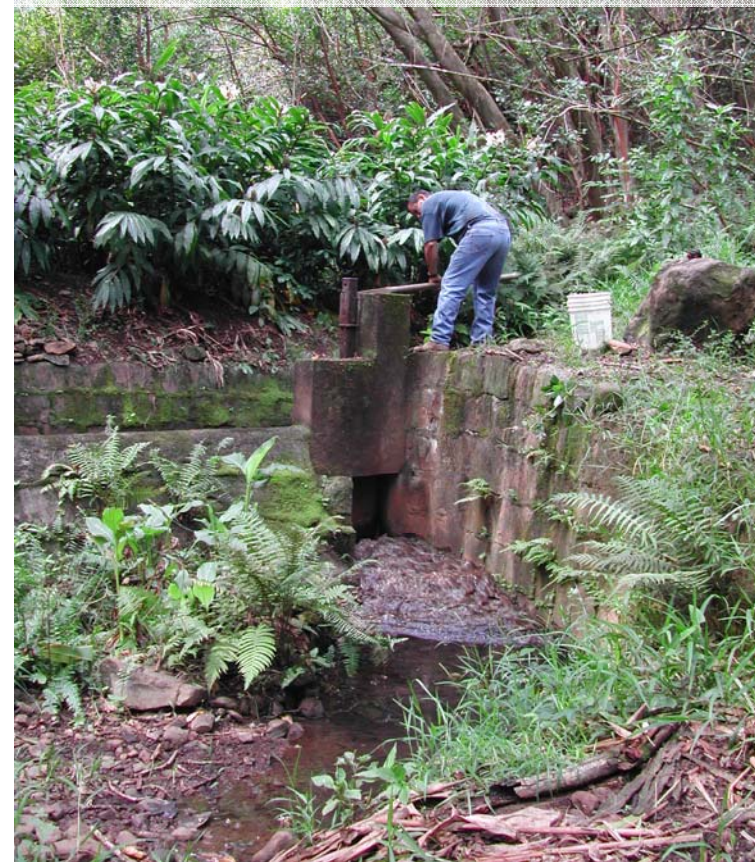
Interim action at Haiku Ditch on Huelo (Puolua) Stream
