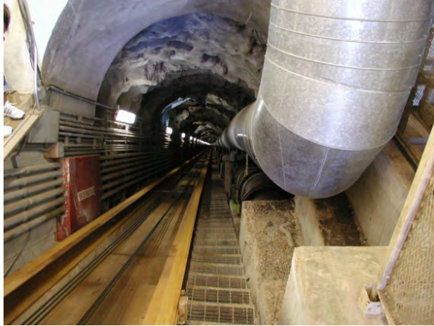
View looking down
