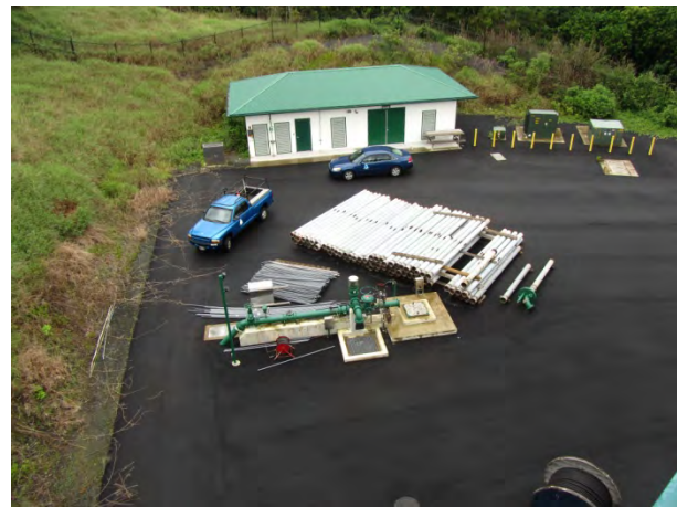
Well pad, column pipe to be installed, & control building
