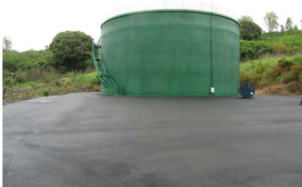
1.0 MG storage tank
