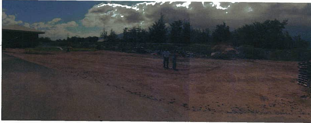
EXISTING MAINTENANCE BUILDING
