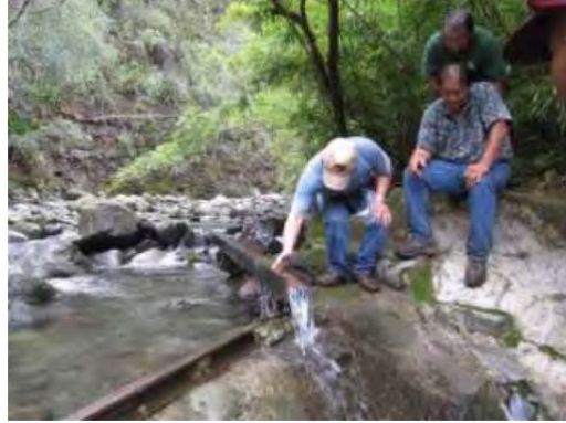
Figure 37: Spreckels Ditch on Waihe'e Stream showing water flowing past the diversion through a small channel. (Image from Dean Uyeno, CWRM, Maui Surface Water presentation at the 1 st Annual Joint State Water Conference)
