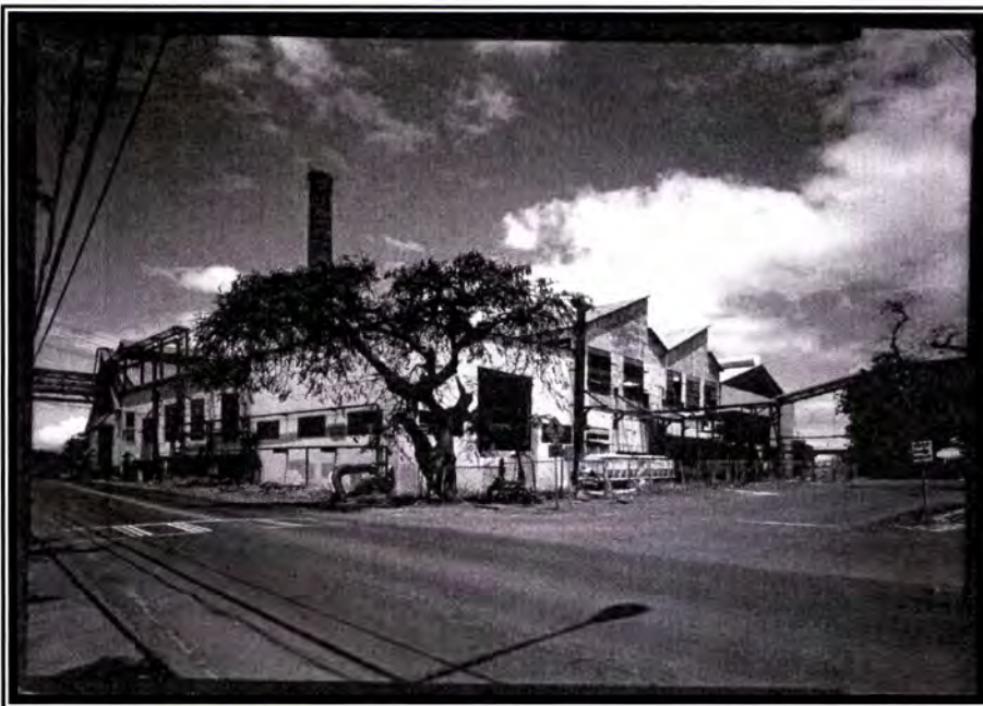
Pioneer Mill in 2005 prior to demolition, Lahaina.
