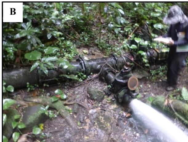
A. Pipeline from development tunnel 15 (HBWS tunnel 1) crossing the right branch of Kalalula Stream at the 1600 ft elev. B. Pipeline from development tunnel 19 (HBWS tunnel 3) discharging 0.47 mgd into Kanewai Stream at the 1450 ft elev.
