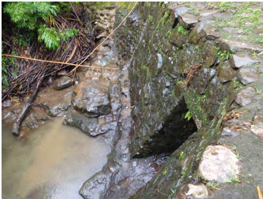
Figure 4-7. Photo shows below the diversion and is taken across the stream. Note there is only a trickle flowing from the gate. (3/12/2009; Tributary name: Kōlea (64003001); PBN: dk003p-017-031209; Surveyor: Kuamo‘o, D.; SBN: dk003n-031209; Lat. (DD): 20.87282, Long. (DD): -156.19005).
