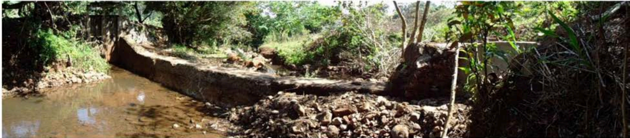
Lawai Stream Dam Diversion 812
