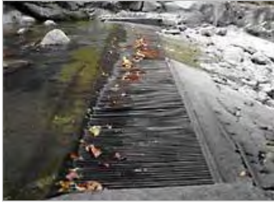
Figure 16. Stream Diversion Channel
