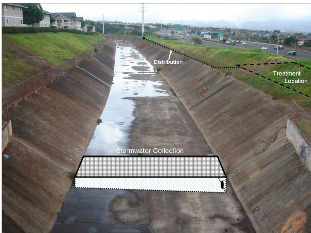
Figure 15. Stormwater Channel Collection Sump Conceptual Design
