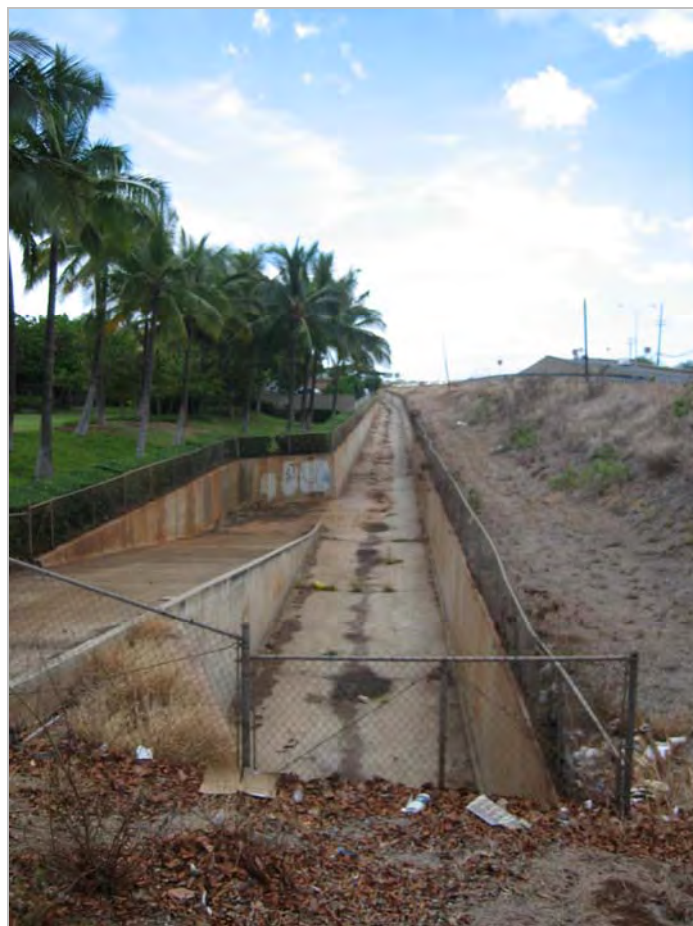
Figure 14. Kapolei Flood Control Channel
