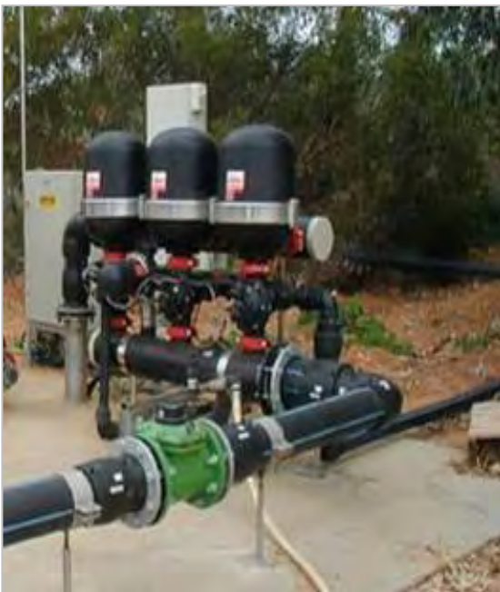
Figure 20. Disc Filtration System
