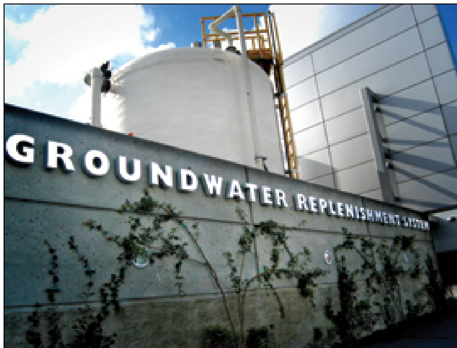
The OCWD uses highly treated recycled water to replenish its groundwater supplies.
