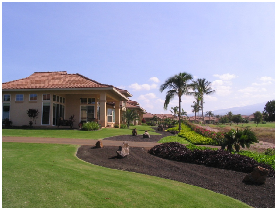
The use of R-1 water for landscape irrigation at single family homes is only approved by the DOH when maintenance of irrigation systems is conducted by contractors. The Hokulani Golf Villas in south Maui is an example of a “managed” irrigation system.
