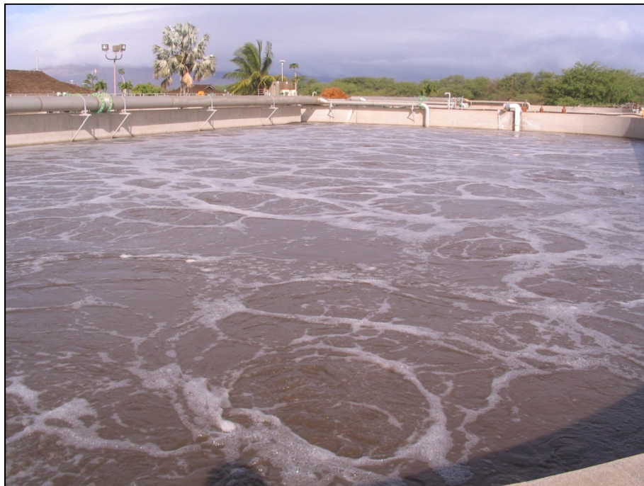
This aeration basin uses activated sludge – one type of secondary treatment method – to treat wastewater.
