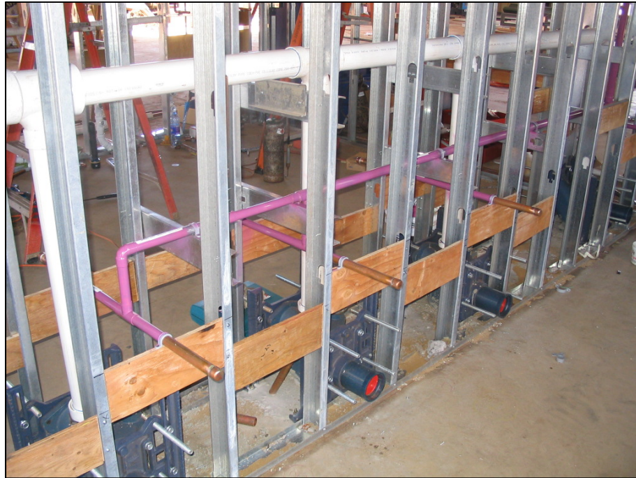
Monsanto installed dual distribution systems within its buildings at its south Maui Piilani farm to accommodate the use of R-1 water for toilet and urinal flushing.
