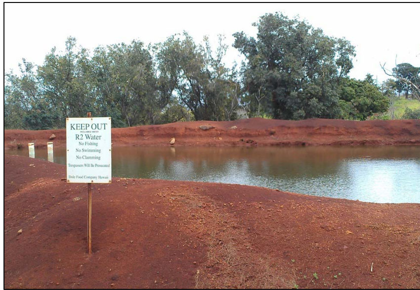
The Dole irrigation ditch conveys water that includes effluent from the Wahiawa WWTP and Schofield WRF.
