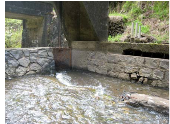
EMI diversion at Koolau Ditch, Wailuanui Stream
