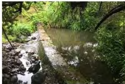
The Lāwa'i Ditch diversion across Lāwa'i Stream from the left bank.
