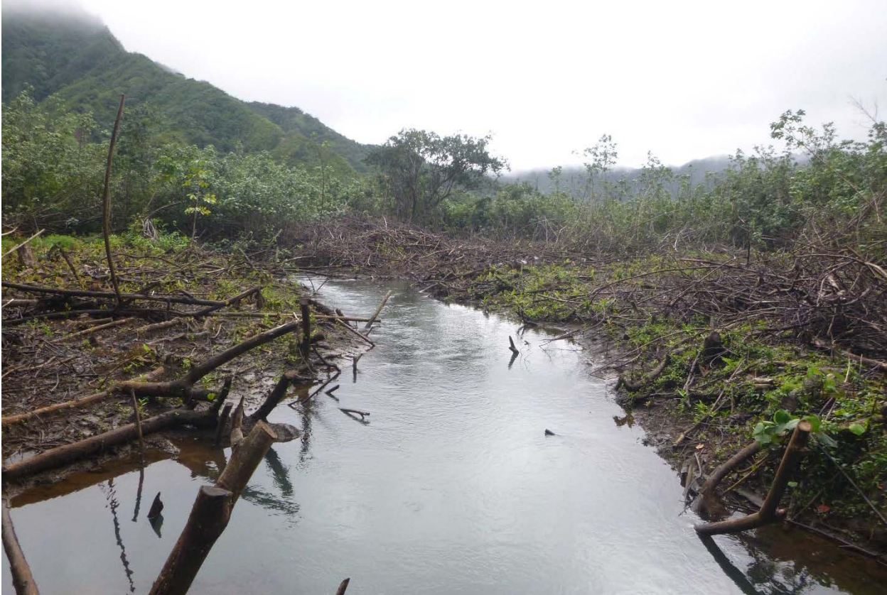
Photo 7. Contracted work on hau clearing (12/23/2016).
