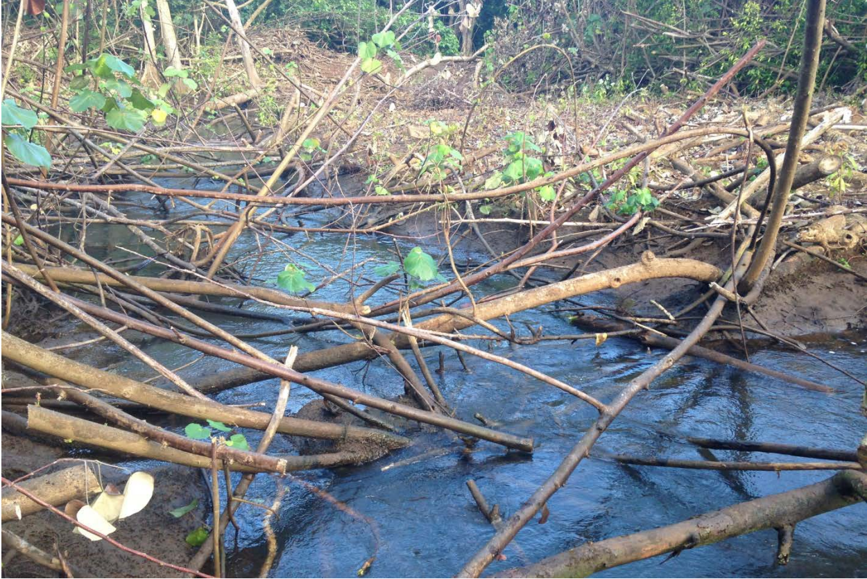
Photo 6. Contracted work on hau clearing (October 2016 – April 2017).
