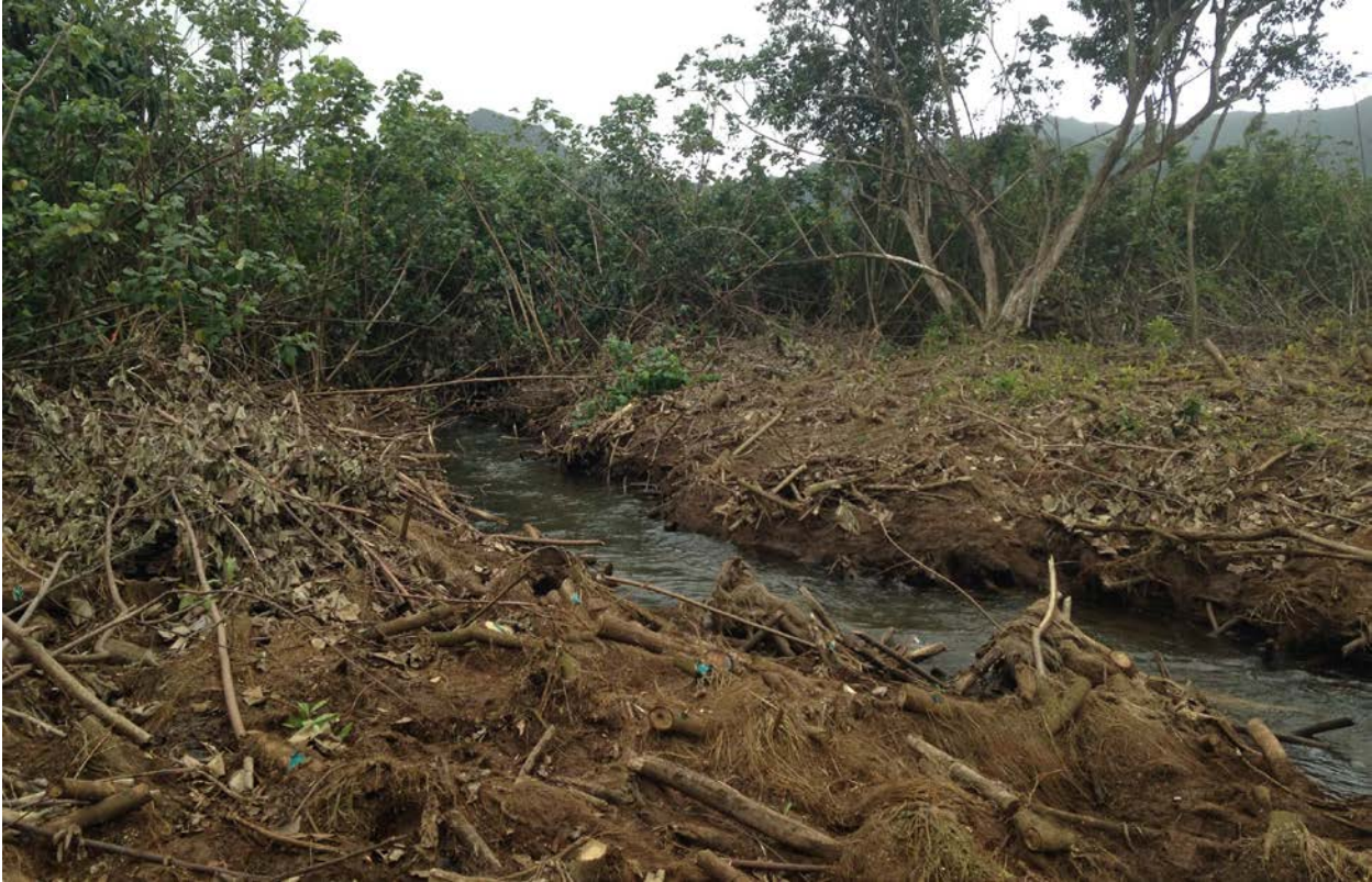
Photo 9. Contracted work on hau clearing (01/31/2017).
