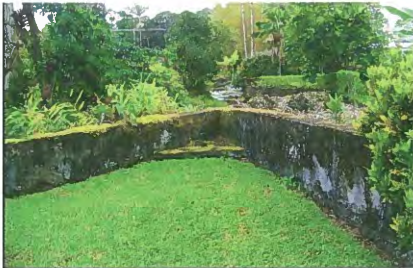
Figure 4. Flood levee along Ainako stream on upstream border of Marsh property. Built circa 1956-58 soon after damaging flood of 1956.
