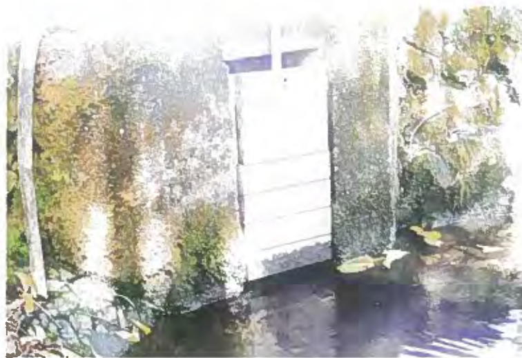
Figure 6. Flood control gate that buffers water flow into the branch stream. In back of the gate is a 14-inch ID diameter four-foot section of concrete culvert. Historic (2 to 4 decade) setting of the gate opening gap (3 ½ -4 inches) provides steady day-to-day water supply while keeping storm flow to non-damaging levels on downstream properties. The present gate, built of plastic wood, replaces the pre-existing steel gate and is set at the historical gap. Station1 in Figure 11.
