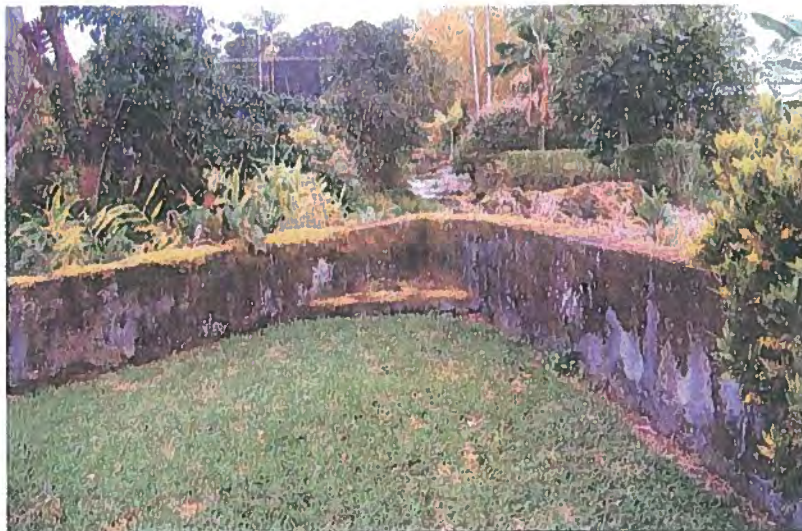
Figure 4. Flood levee along Ainako stream on upstream border of Marsh property. Built circa 1956-58 soon after damaging flood of 1956.
