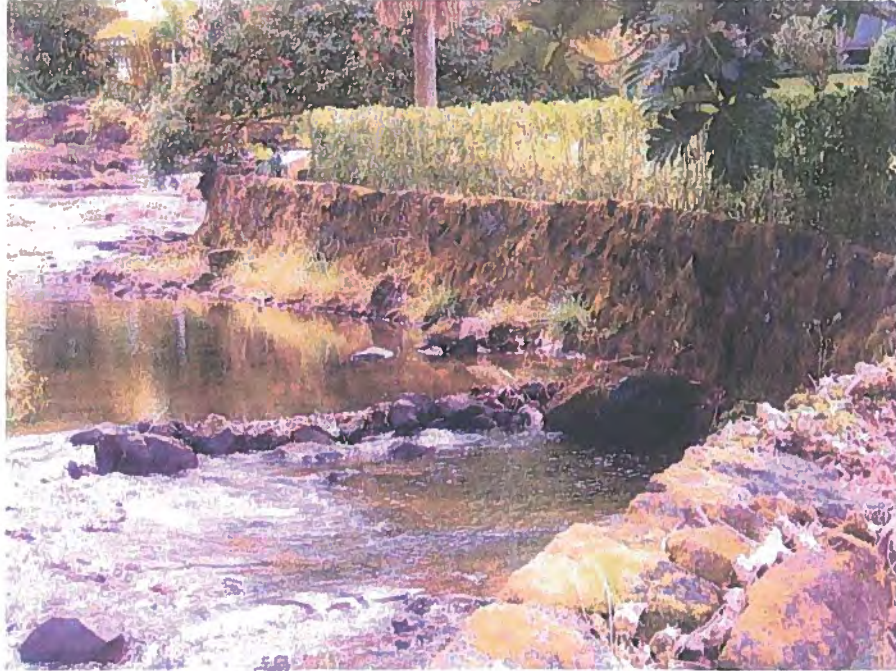
Figure 5. Levee embankments along the Ainako stream Weight property margin.
