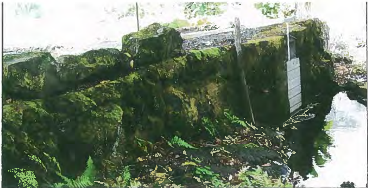
Figure 7. Flood control gate and reinforced embankment at origin of branch stream.
