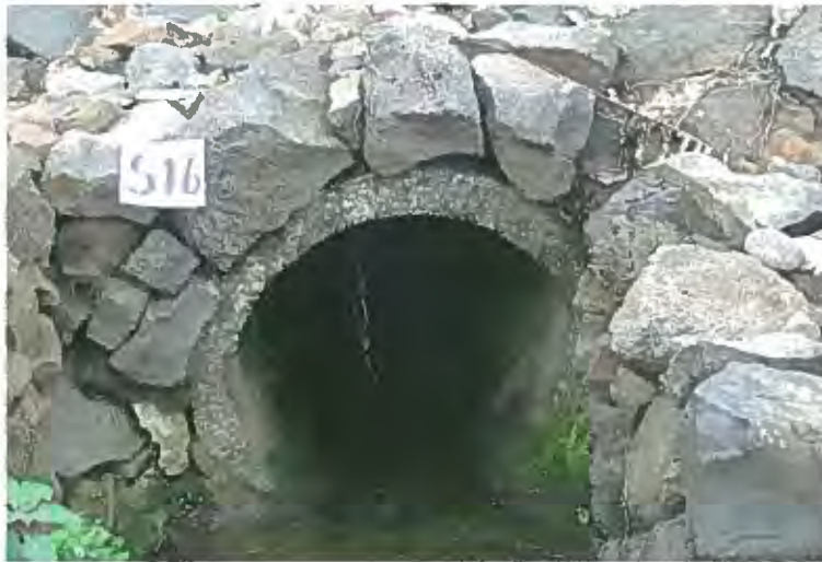
Figure 26. Station 16 of branch stream looking downstream at culvert that passes under Kokea Street.
