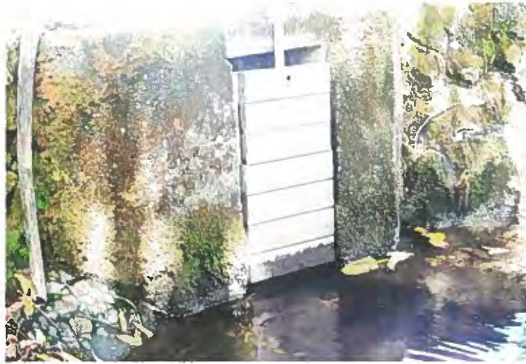
Figure 6. Flood control gate that buffers water flow into the branch stream. In back of the gate is a 14-inch ID diameter four-foot section of concrete culvert. Historic (2 to 4 decade) setting of the gate opening gap (3 ½ -4 inches) provides steady day-to-day water supply while keeping storm flow to non-damaging levels on downstream properties. The present gate, built of plastic wood, replaces the pre-existing steel gate and is set at the historical gap. Station 1 in Figure 11.
