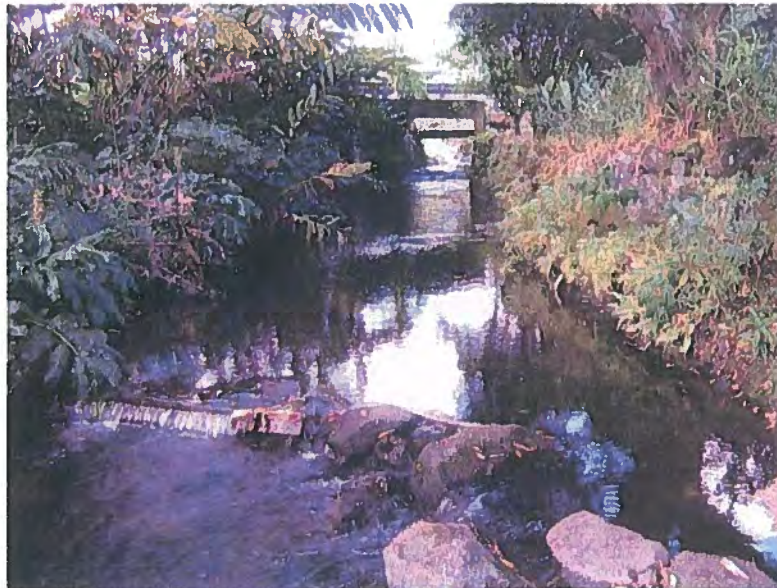
Figure 9. Diversion dam (in left foreground) that raises Ainako stream level to divert water into the branch stream culvert. Ainako Avenue bridge is seen in background.
