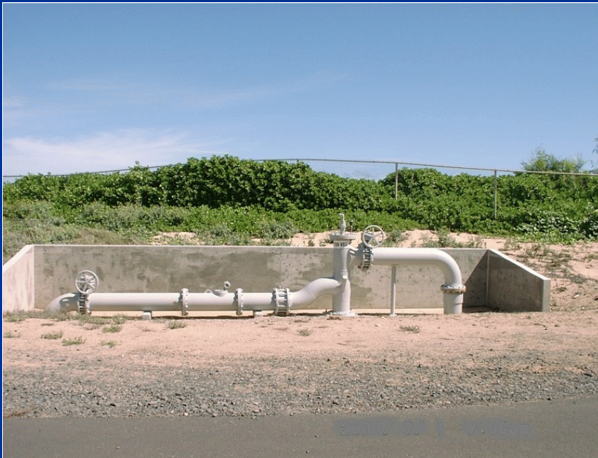
Disposal via injection wells (69% or 7.9 mgd)
