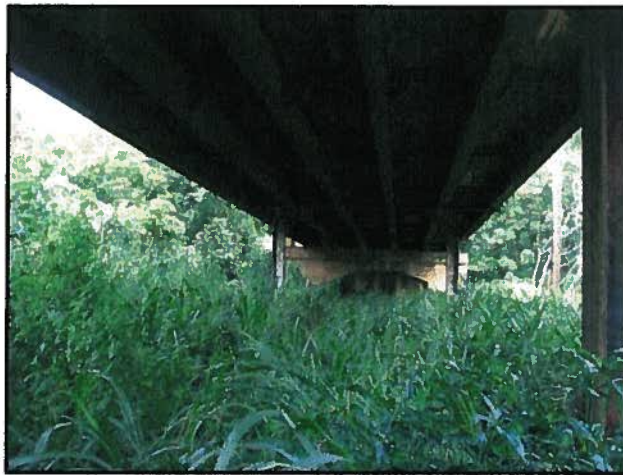
Below existing deck looking east
