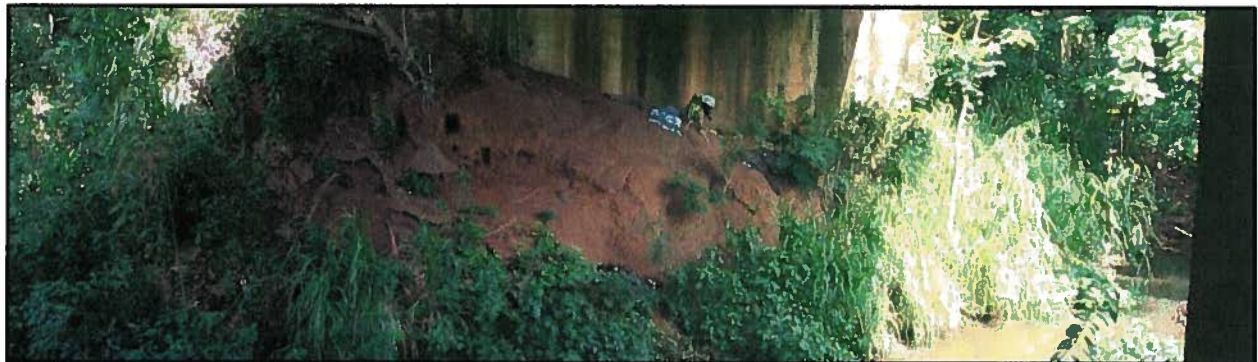
Existing east bank abutment
