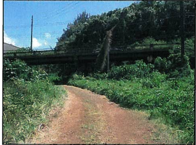
Lihue Mill Bridge looking south
