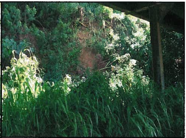
Vegetation on the west bank upstream
