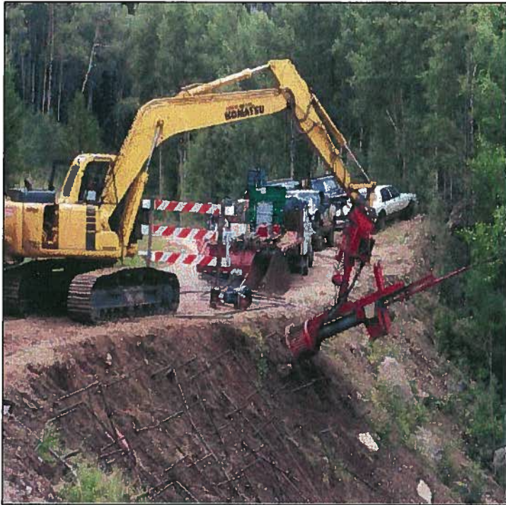
Examples of soil nail installation.
