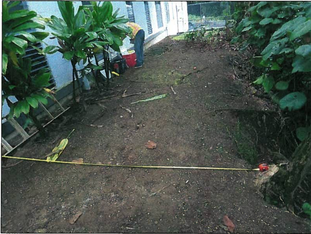
Proximity of the Riverside Apartment building to the edge of the embankment.
