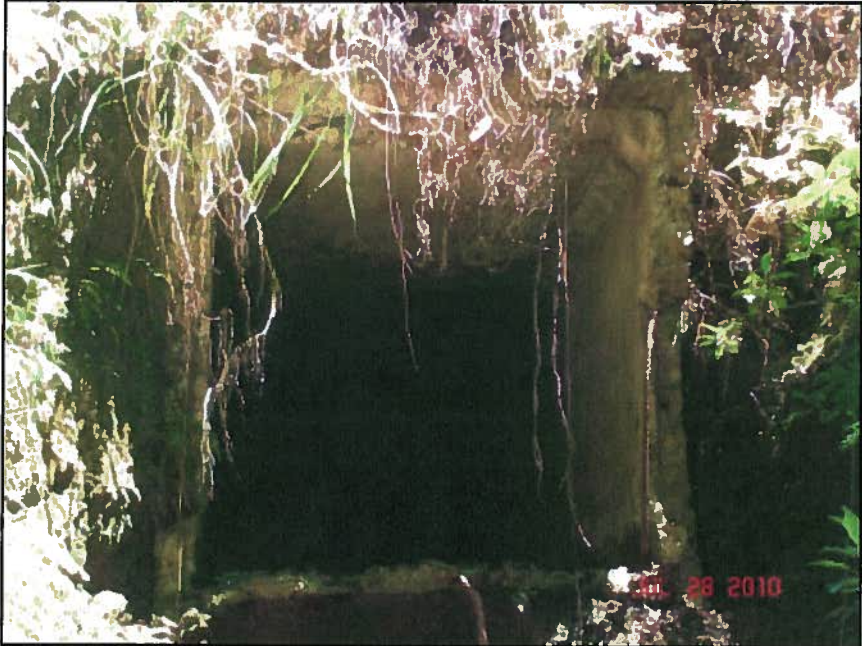
Damaged Box Culvert (top photo) and Scour Pool (below photo).
