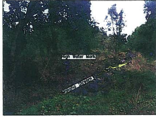
LOOKING DOWNSTREAM AT LEFT BANK
