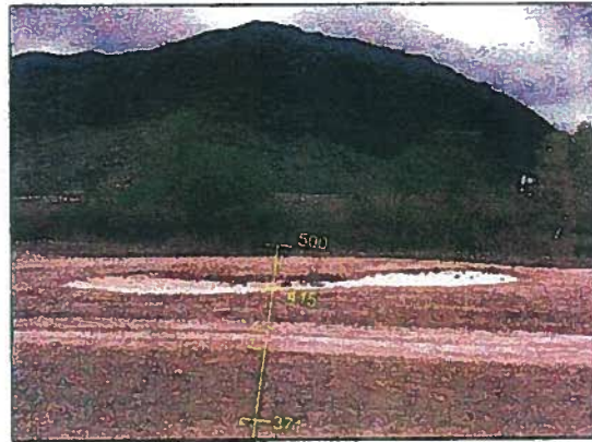
ALIGNMENT 3+71 FACING NORTH
