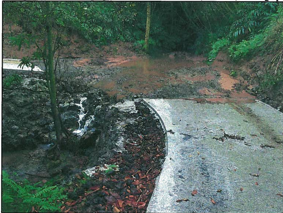
After photo of fill and riprap to streambed and banks (after rain) looking upstream.
