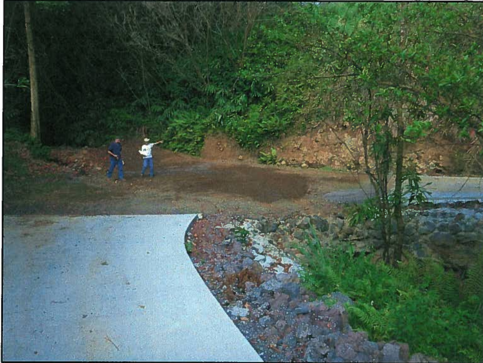
After photo of fill and riprap to streambed and banks (before rain) looking upstream.
