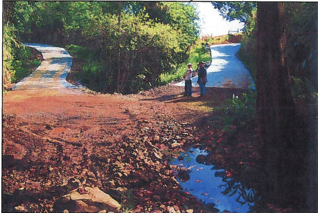
After photo of fill to streambed and banks (looking downstream).
