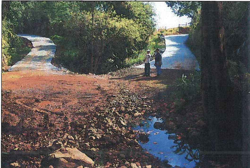
After photo of streambed and banks (looking downstream).
