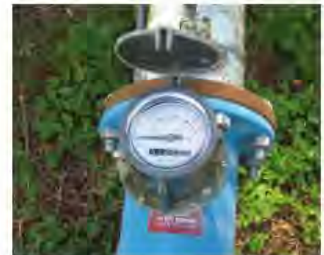
Water meter with totalizer. (HAWAII Well Construction & Pump Installation Standards)
