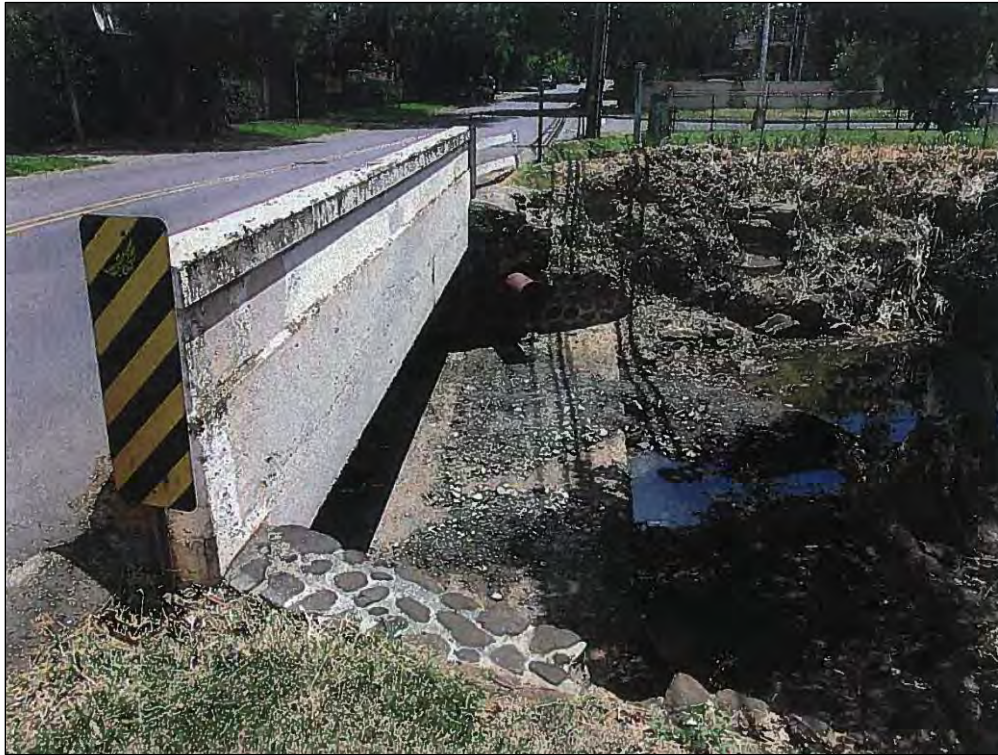
Photo No. 1: North View, Mauka Side.
