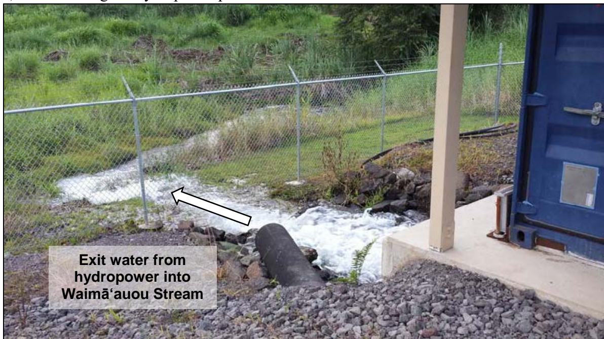
d) Water exiting the hydropower plant in Waimā'auou Stream.
