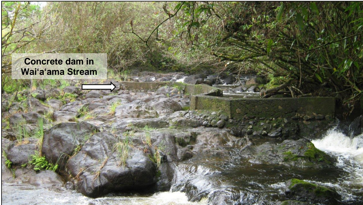
a) Upper concrete dam leading into the flume looking upstream.
