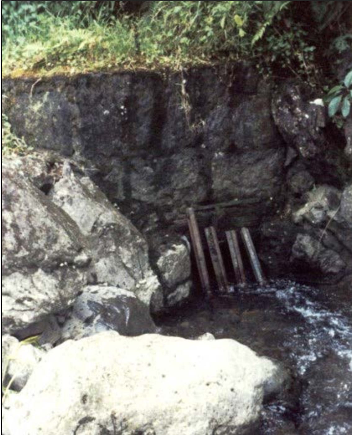
Photo 5. Lalahai #3 intake at Hauoli Ditch (K-27) (1989).
