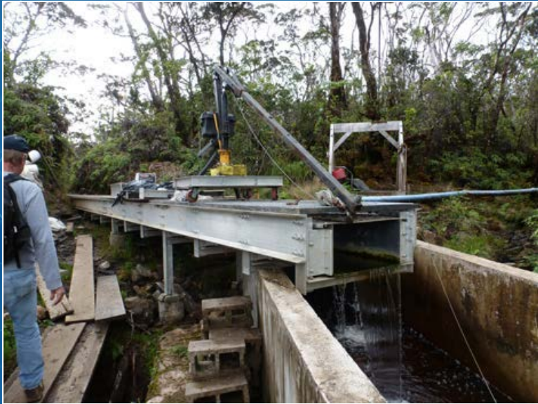
Waikamoi Flume Repair/Replacement Upper Kula Water System, Maui $8,362,760 DWSRF project
