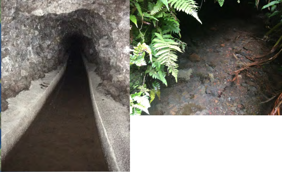
Honokōwai: Tunnel 20-B
