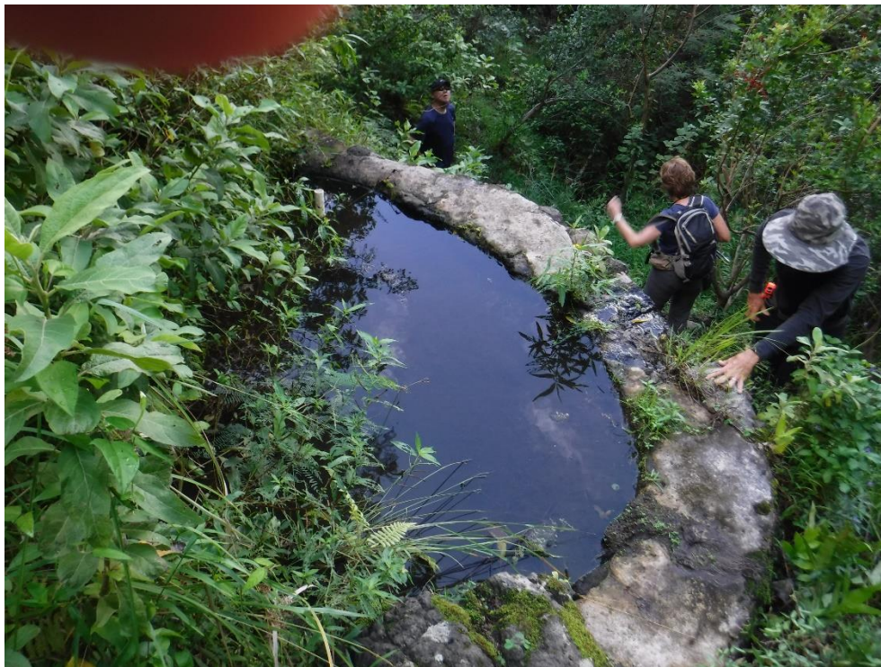
Div 655 Top View : Approximate arc length is 19 feet. Pool is filled with silt, one foot below water surface.
